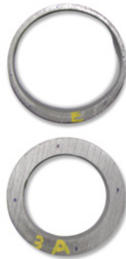
Fig. 2. Single-phase FAC caused the substantial wall thinning shown. Source: ChemTreat.
